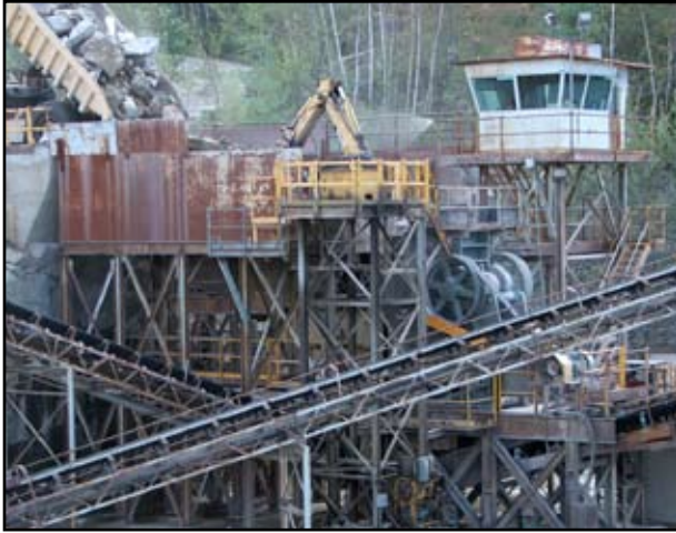
50-ton haul trucks deliver a consistent diet of stone to the new jaw.
